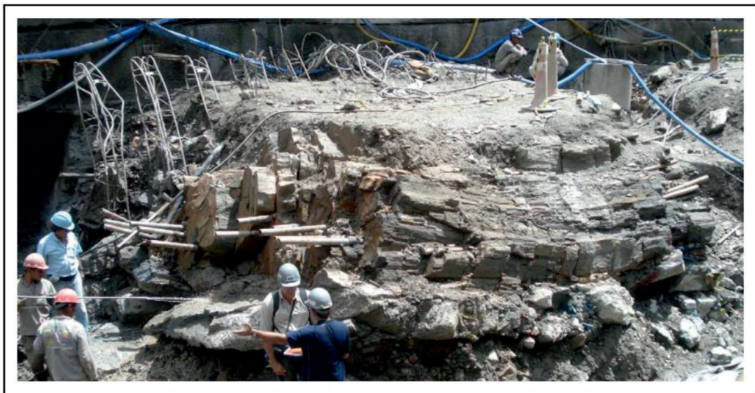
Figure 23 – Severely overloaded vertically, lattice girders demonstrate insufficient strength
