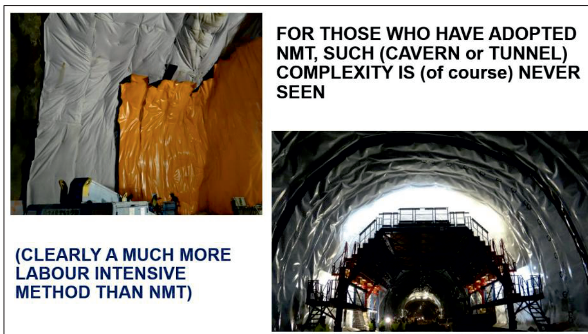
Figure 19- The remarkable labour-intensive NATM if used in a cavern instead of S(fr)
