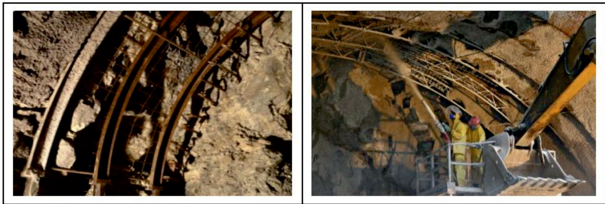
Figure 20 - Steel ribs (left) in an Ecuador HEP, and 32 mm × 25 mm × 25 mm lattice girders in a Brazilian metro station cavern (Barton, 2008)
