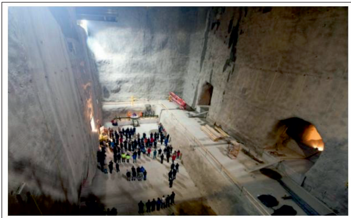
Figure 33 - Construction of large machine hall in Austria using NMT
